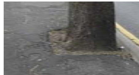
Mature sycamores on Monks Road, causing the pavement to bulge.
