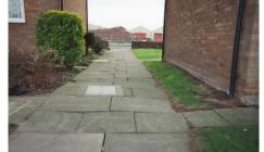
It is bad enough simply having to walk on this paving, especially when it is wet and small jets of water shoot upwards – imagine pushing a pram or using a wheelchair on this surface.
